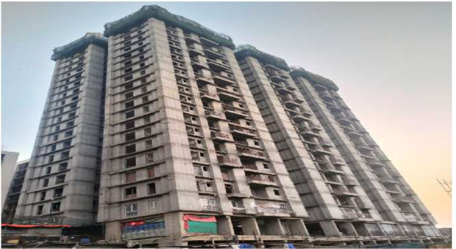
TOWER 2 :: SLAB AT 23 rd FLOOR LEVEL IN PROGRESS
